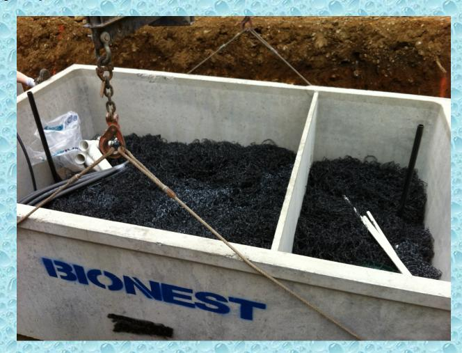
TYPE 3 - Package treatment unit followed by a ultraviolet light unit to kill bacteria, or additional thickness of engineered sand. Septic field size can be 60% smaller. Design by Professional only.
